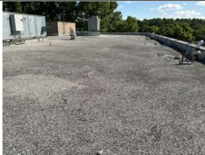
8 - ROOF (OLD BUILDING)
