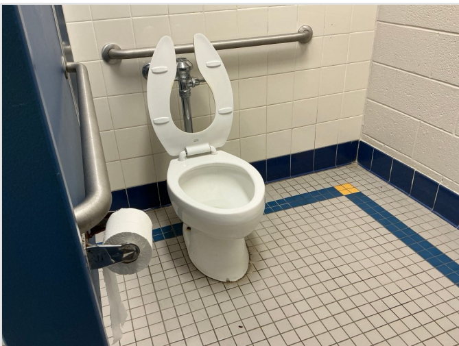
TOILET STALL OVERVIEW
