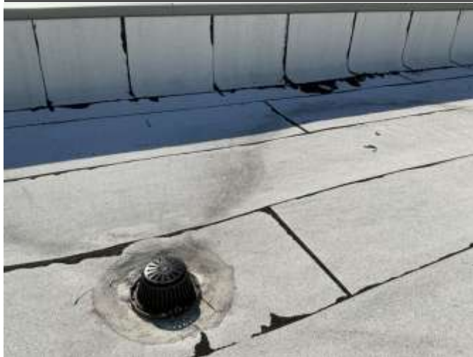
7 - ROOF (NEW ADDITION)
